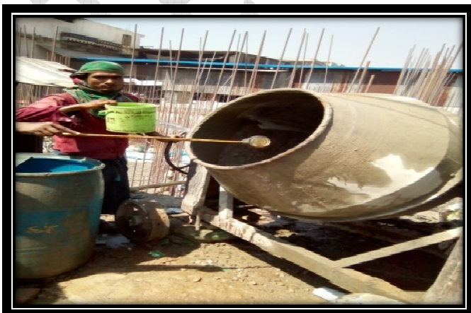
ETP Concrete Casting Using Best Con-WL
