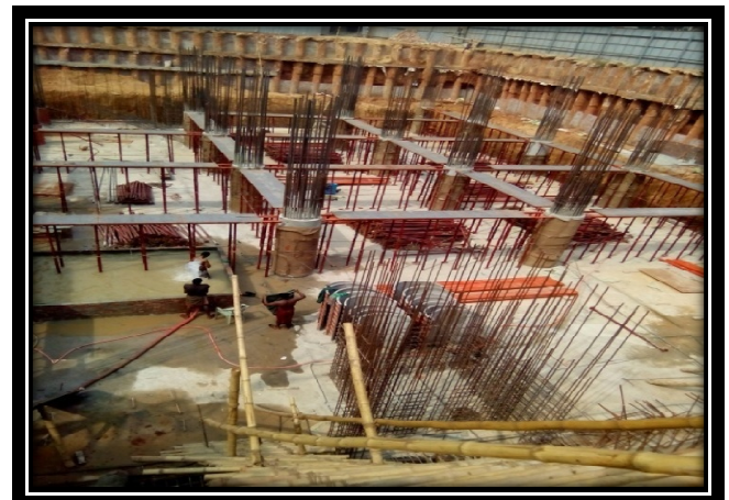
Using Best Con -WL for Basement mat & Returning wall
